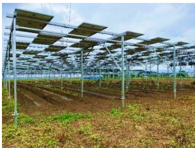
OSG solar power plant where corn sprouts are growing
