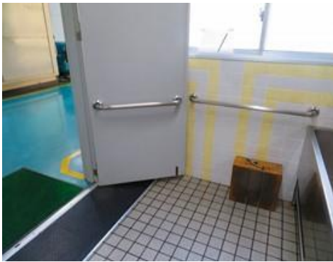
Barrier-free for preventing tripping and falling (Yana Factory)
