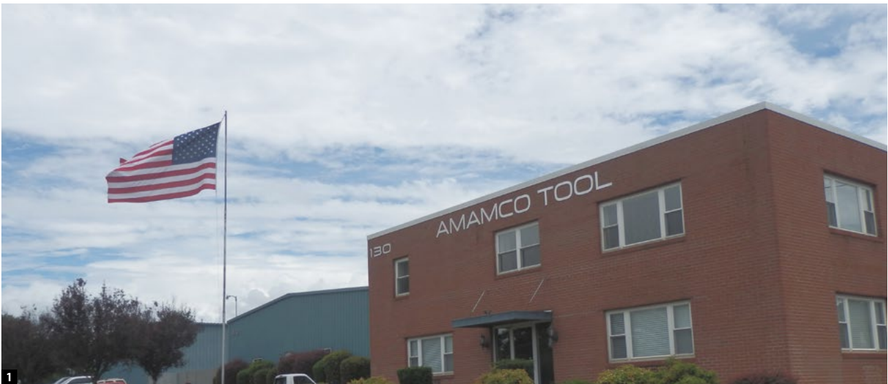
1. AMAMCO Tool in Duncan, South Carolina, USA. AMAMCO is well known for manufacturing combination drills, countersinks, counter bore and high-quality reamers.
