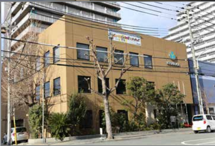
Yoshioka Kogyo's headquarters in Kobe, Japan.
